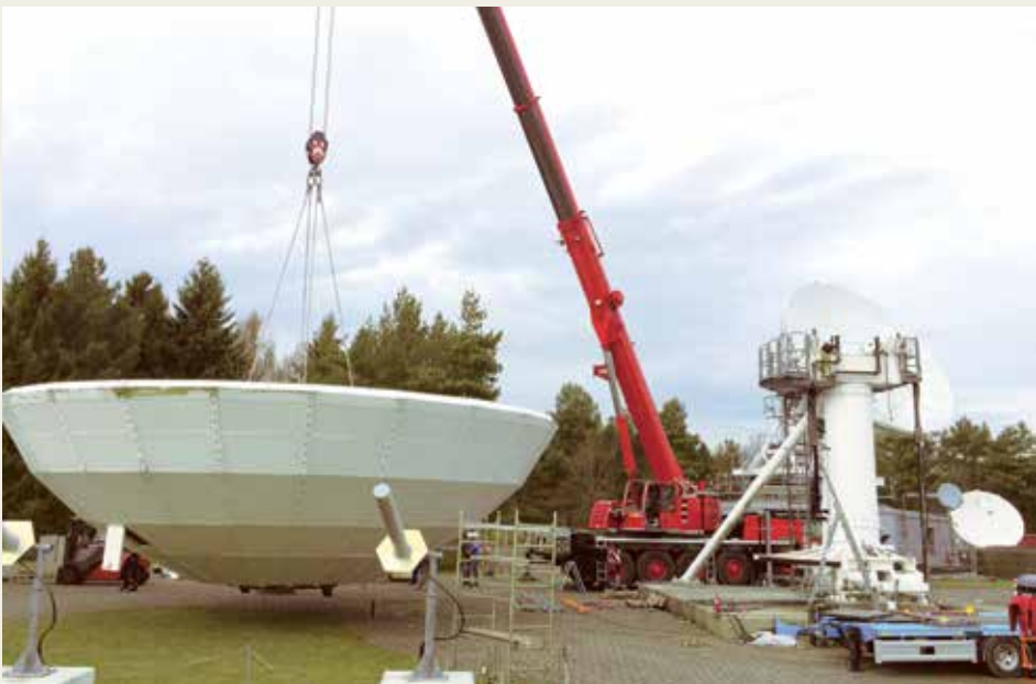
Dismounting of one Meteosat backup antenna in Usingen for shipment to Cheia
